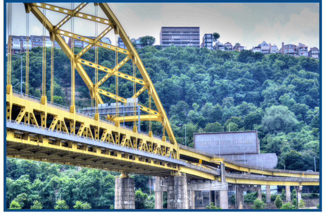
Fort Pitt Tunnel
